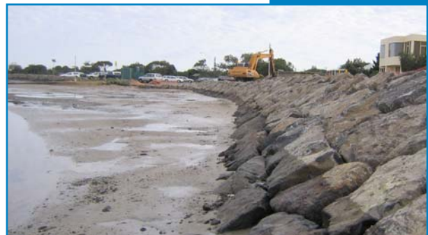
Above: Barwon River Project under construction
