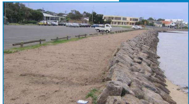
Above: Barwon River project finished
