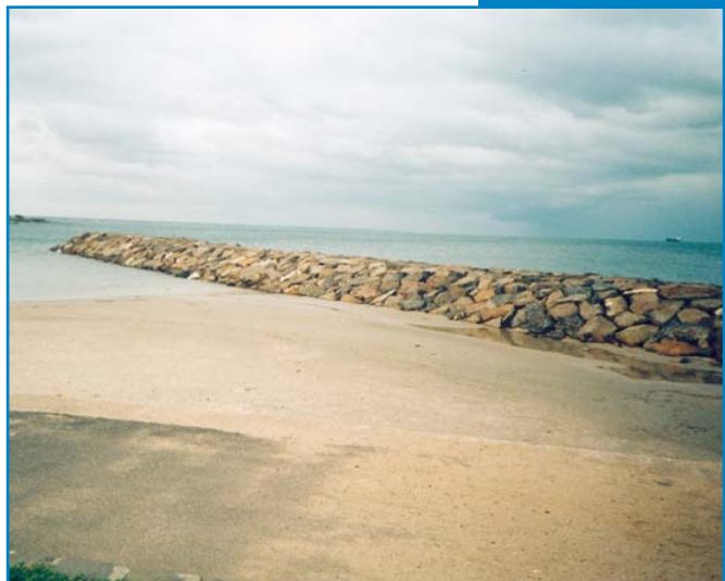
Above: after construction
