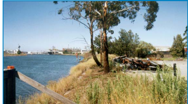
Above: before construction – Maribynong
